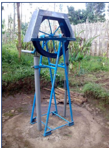
Figure 3.1 Good rope pump, but installed below ground level, with no drainage or spout
