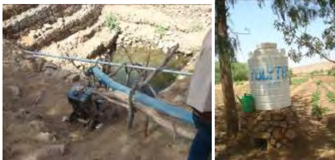
Water is pumped from the protected hand-dug well by a diesel motor into a small water tank
