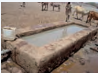
Comparing technology choices in cattle troughs: metal sheet troughs are easier to move around and carry, in comparison to concrete ones, which are sited.
