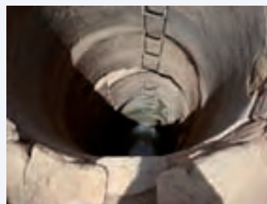
Twin hafirs feed the nearby water yard, through wells. There used to be a storage tank, but this has gone into disuse due to the conflict. There is currently no control over access. Disused wells are guarded against people or animal falling in and the water is not treated.
