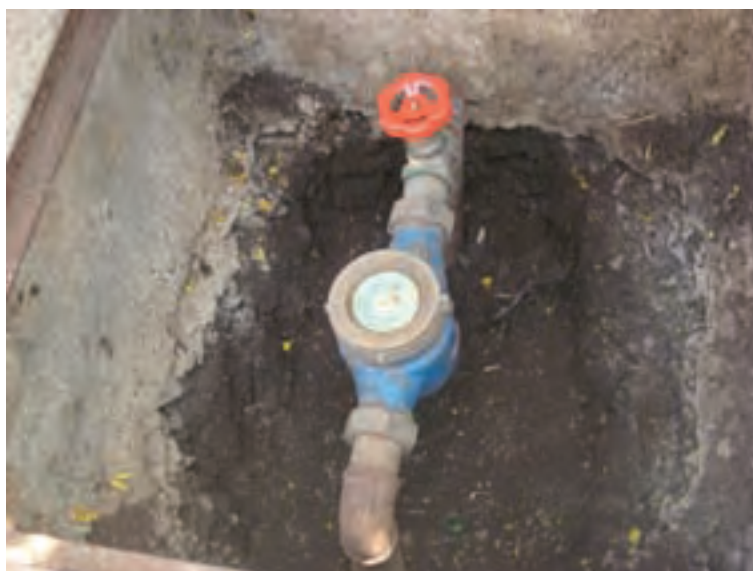
Metering is key in aiding cost recovery and financial sustainability in Kabuku.
