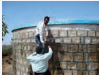
System is a motorised pump which feeds storage tanks, with distribution points that are fed by gravity. The functioning distribution points are the taps where water is collected for domestic use.
