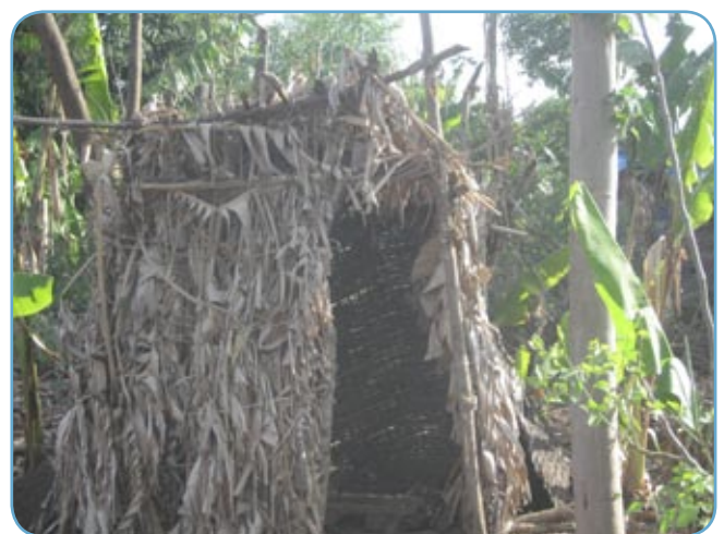
Latrine from local materials, SNNPR
