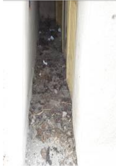
Case 2. School toilet
